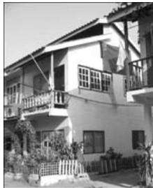
These 2.5-story rowhouses at Ruam Samakee offer 110 m<sup>2</sup> of living space, and were built by the community's own construction team for an average of 310,000 Baht (\$8,857 per unit). Average construction cost was 2,818 Baht (\$81) per m<sup>2</sup>.
