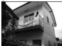
These 2-story rowhouses at Klong Bang Bua offer 100 m<sup>2</sup> of living space, and were built in phases by the community's own construction team for an average of 322,000 Baht (\$9,200) per unit. Average construction cost was 3,220 Baht (\$92) per m<sup>2</sup>.
