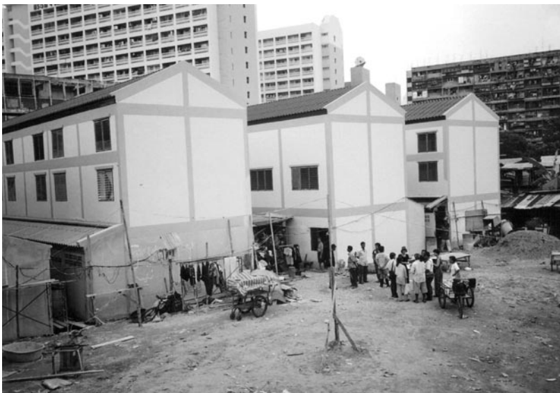
Photos 1 and 2: Bon Kai before and after reconstruction
